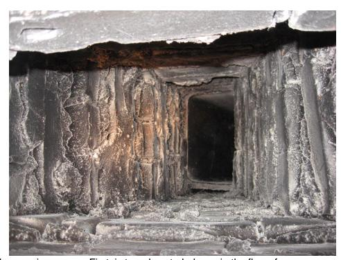
chimney that is done for three main reasons. First, is to reduce turbulence in the flow of combustion gases. Second is to prevent combustion residue or smoke from leaking or accumulating in crevices or parts of the chimney.
